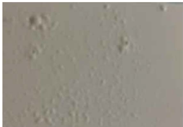
An example of blistering and discoloration caused by drying at a too rapid rate
